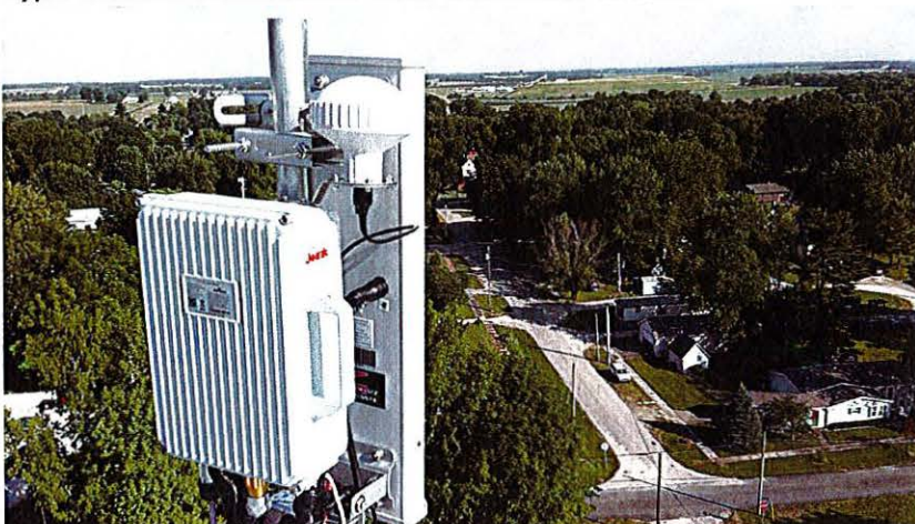
Type 4: 3.5GHz Baicells LTE radio with sector antenna
