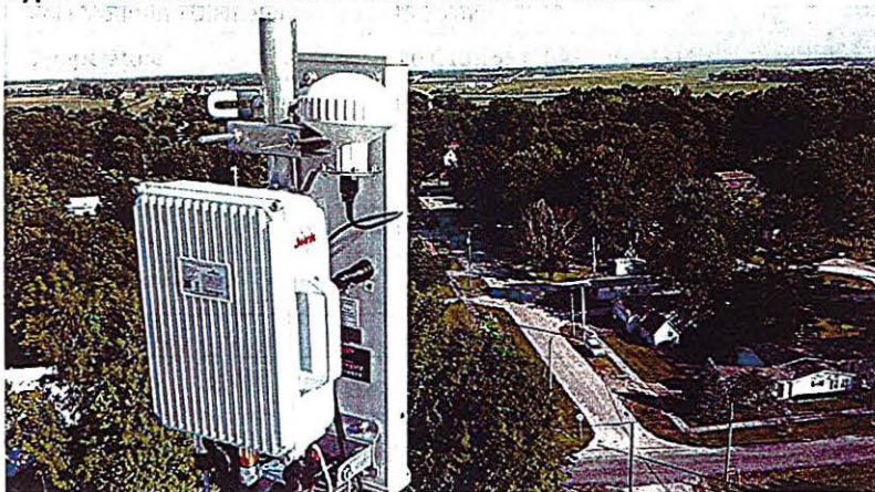
Type 4: 3.5GHz Baicells LTE radio with sector antenna
