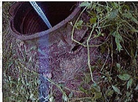
Hole in Frame (allows inflow)
