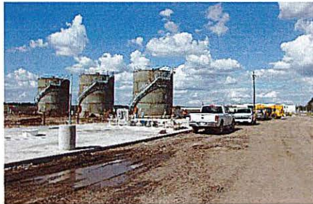
Construction of the three vertical steel tanks is near completion, with next steps including paint and plumbing service lines.
