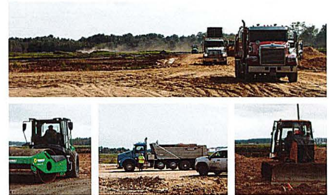
Construction is progressing well on this 60 acre site managed by the joint venture of Barnhill Contracting and TA Loving Company.
