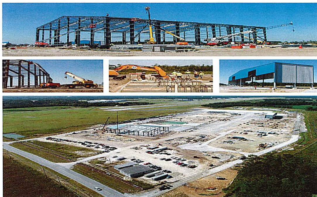
The Barnhill Contracting and TA Loving Company, Joint Venture, continues the momentum of the construction of the C-130 project and its 60-acre site.
