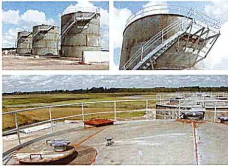
Construction of the three vertical steel tanks is near completion, with next steps including paint and plumbing service lines.
